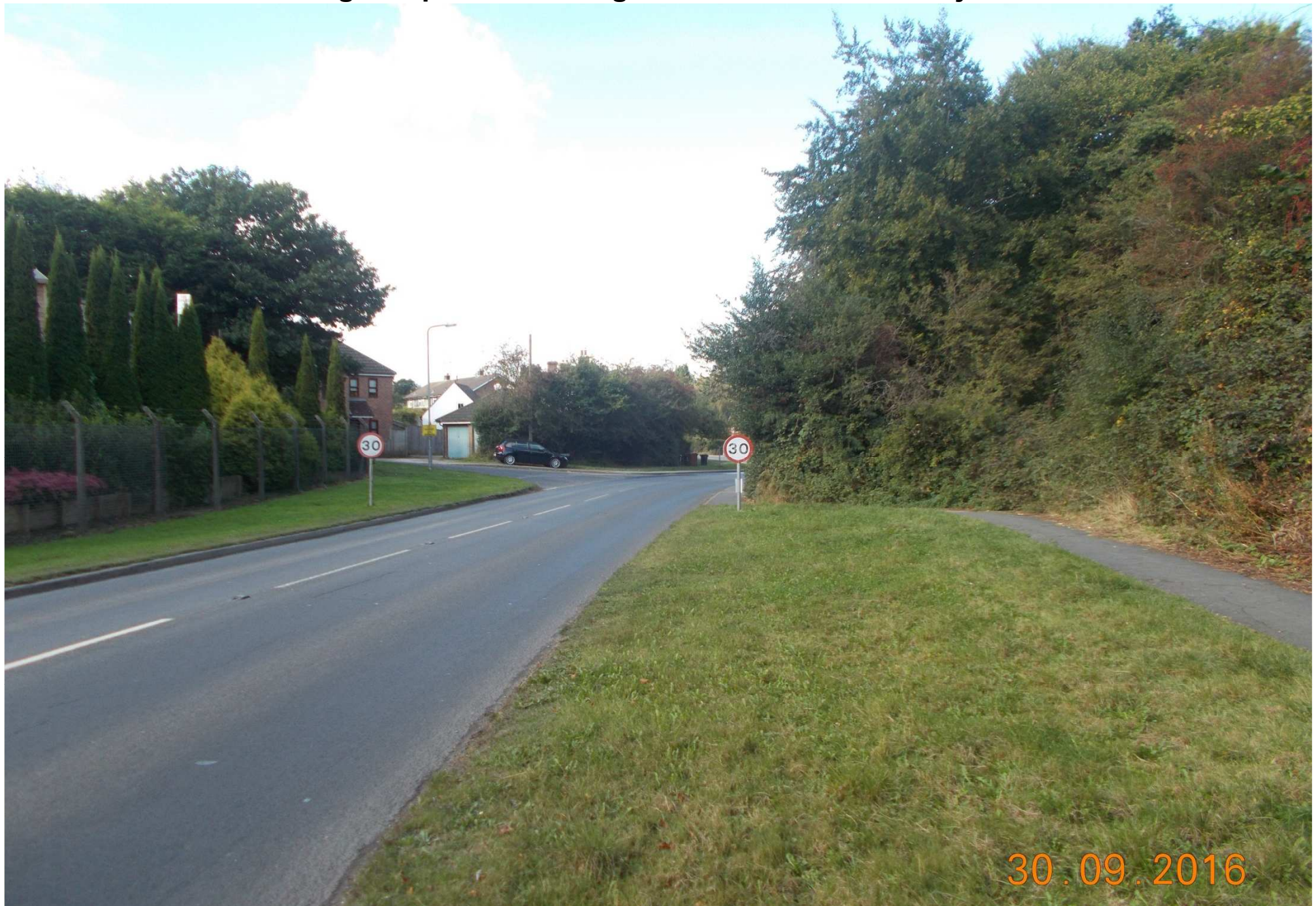
View of the existing 30mph terminal signs near the Mottins Hill junction
